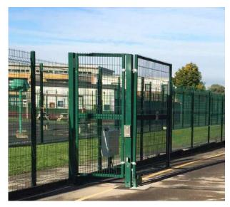
Typical style of new pedestrian gates to G1, G4, G5, G7 & G8 - All gates to be 2200mm to match fence height - width as per drawing ref: 2335\_T\_003
