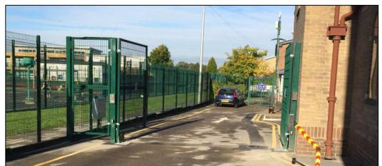
Typical style of new double vehicular gates to G3 - Vehicular gate to be 2200 x 4000mm as per drawing ref: 2335\_T\_003 to enable emergency vehicle access.
